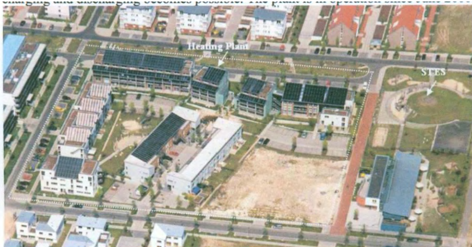
Fig. 2-30: CSHPSS in Hannover (source: Gockell)
